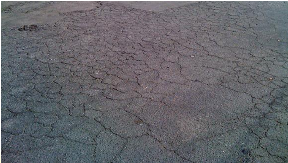
Fig. Alligator Cracking
