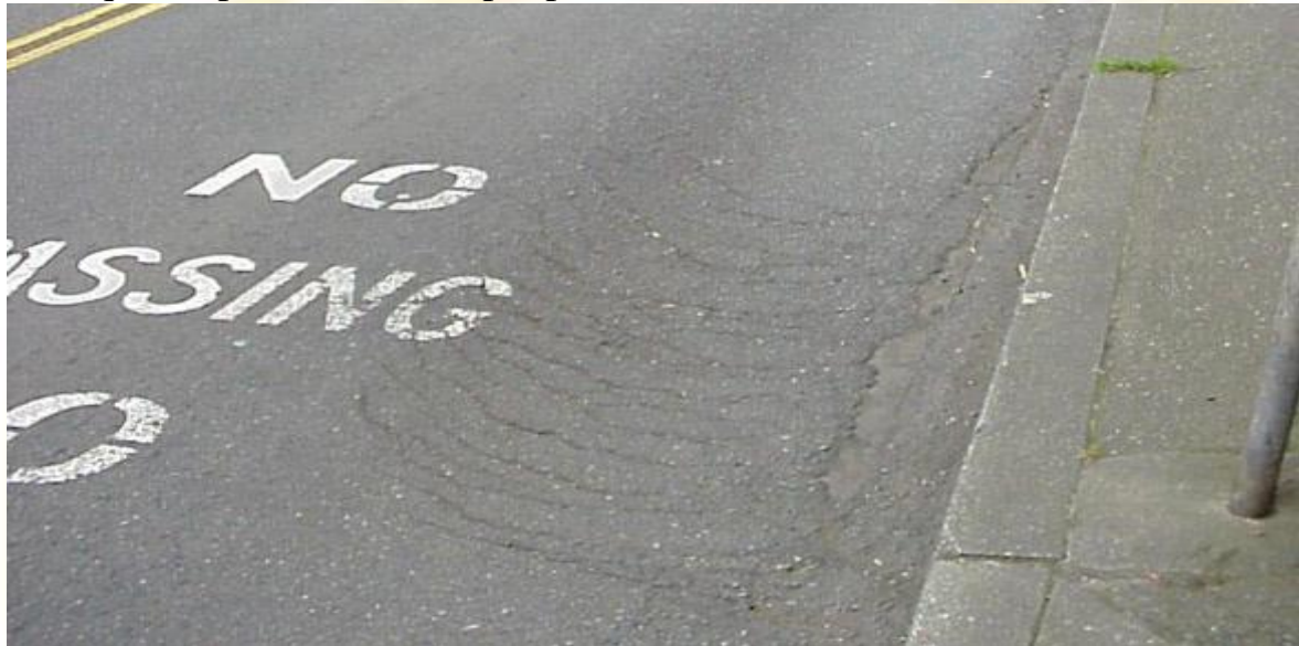
Fig. Slippage Cracks
