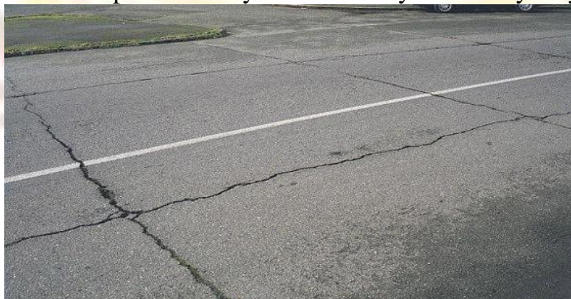
Fig. Joint Reflection Cracks
