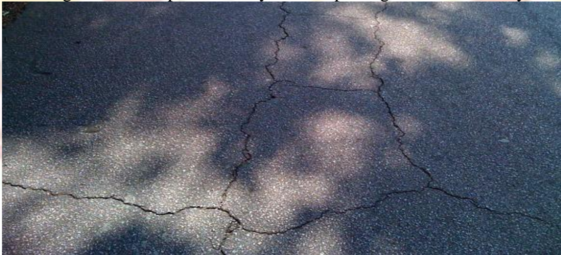
Fig. Block Cracking
